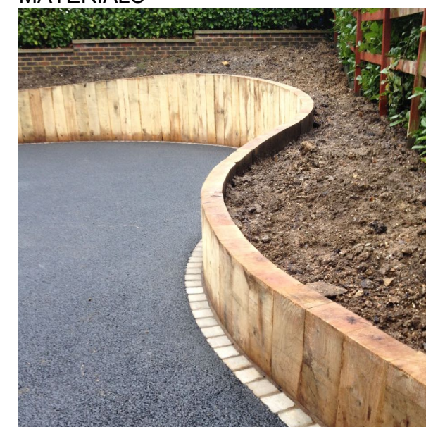
Railway slipper retaining wall
