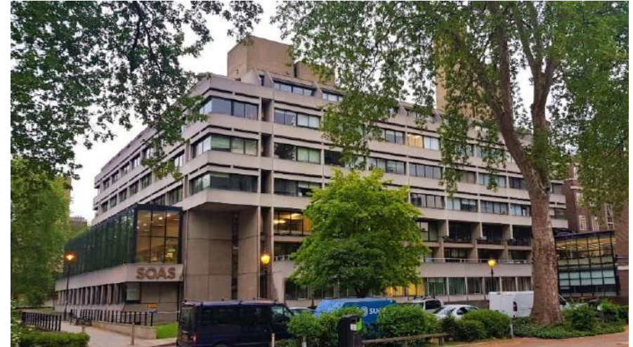
Fig. 02 - Philips Building, Northern and Western Elevations
