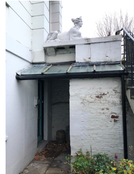
fig 11. Side of existing coal store beneath the entrance way
