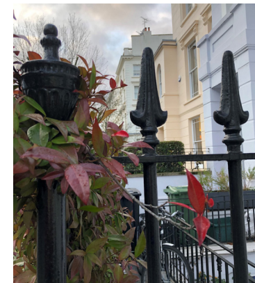
fig 13. New balustrade across the top of the existing wall shown in fig. 12 will match the adjoining property (shown above)
