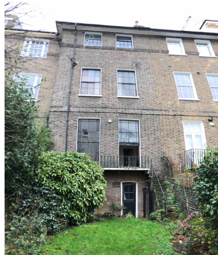
fig 5. Existing rear facade showing minimal access to garden from lower ground floor
