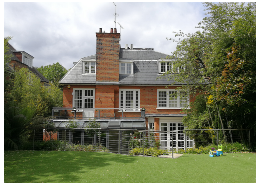
View from the back of garden towards the building and existing steps
