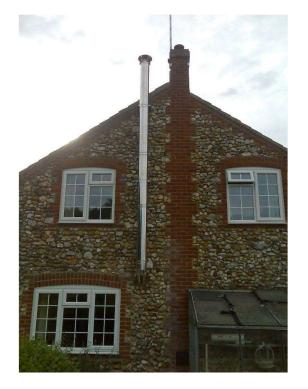
For this proposal, to ensure that they are aesthetically acceptable in the context of the Property and the Conservation Area, the steel flue will be powder coated to match the colour of the existing brickwork that the flue will run along. The RAL code and colour is as follows:
