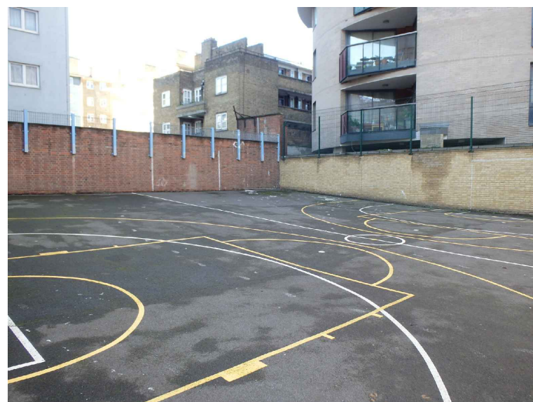
View 4. Existing ball court - visible slope
