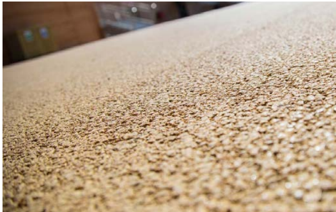
Buff colour macadam to the ramp and the outdoor gym
