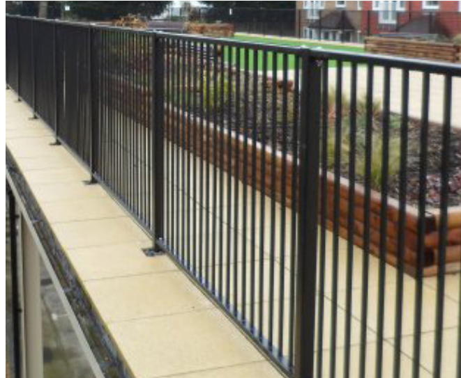
Flat top metal railing to the outdoor gym
