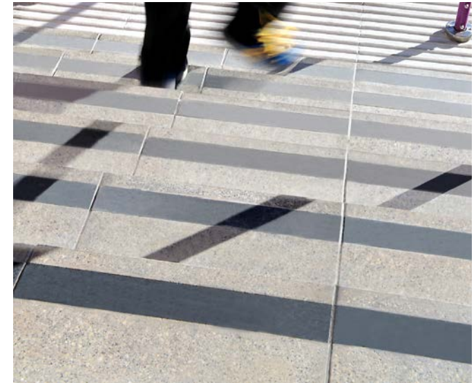
Concrete slab stairs
