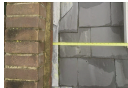
8- Dimension between panel and parapet as built
