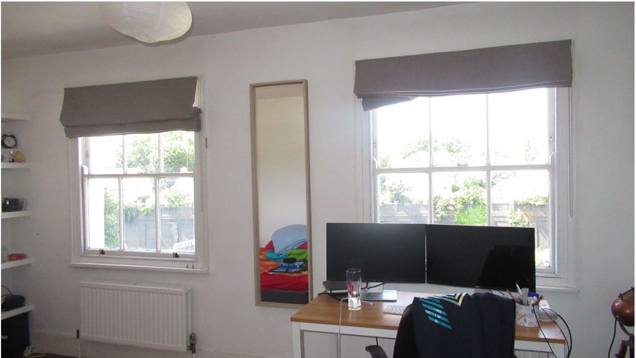
Figure 5: Internal view of windows at third floor
