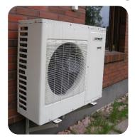
Air Source Heat Pumps (ASHP) employ the same technology as Ground Source Heat Pumps (GSHP). However, instead of using heat exchangers buried in the ground, heat is extracted from the external ambient air.
