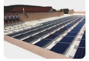
Solar photovoltaic (PV) cells generate electricity from the sun's energy. Solid PV panels can be either roof or façade mounted (although solar modules fitted on a south facing façade have only 75% the output of roof mounted modules).
