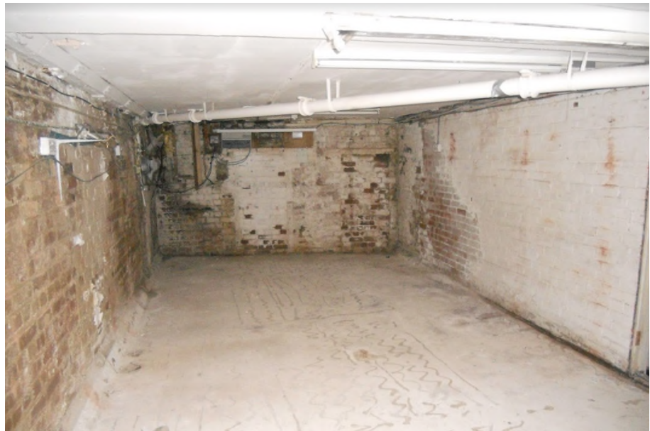
Existing vacant basement space
