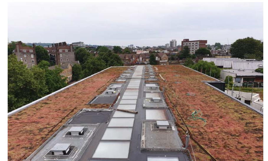
Existing green roof with corridor rooflights
