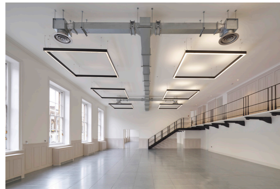
Ground Floor (South) Office - 183
