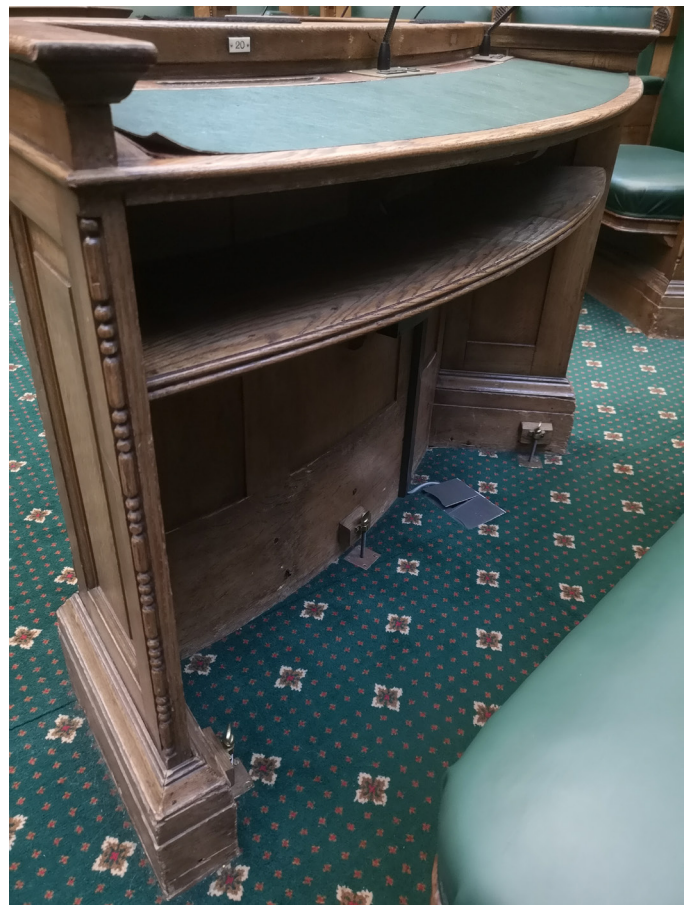
Existing removable bench to provide wheelchair accessible seating
