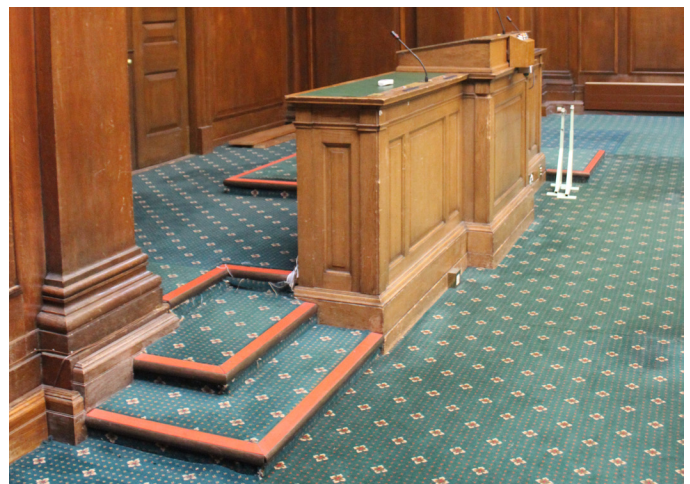
Existing dais arrangement with stepped access and split-level platform
