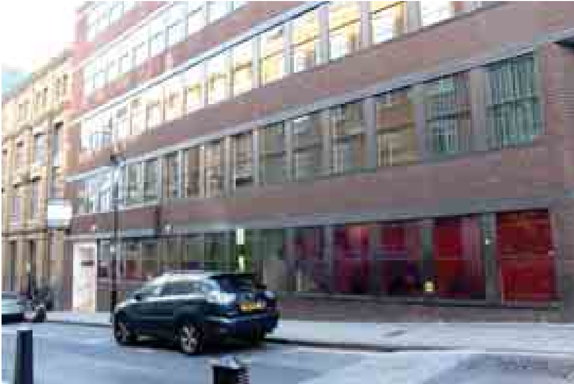
Fig 13 View looking south-east, showing the northern side of the existing building within the site (MOLA site visit 03/11/2017)
