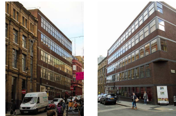
Existing building at 20-23 Greville Street.
