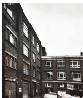
Photograph showing rear elevation of 20-23 Greville Street.
