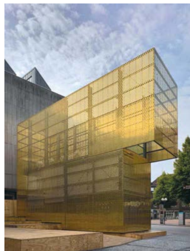
Fig. 134. Information centre - Switch.
