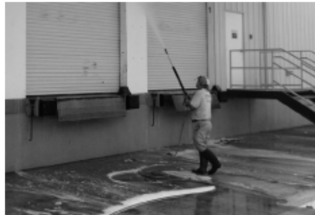
Fig. 105. External Cleaning - Pressure washing the outside
