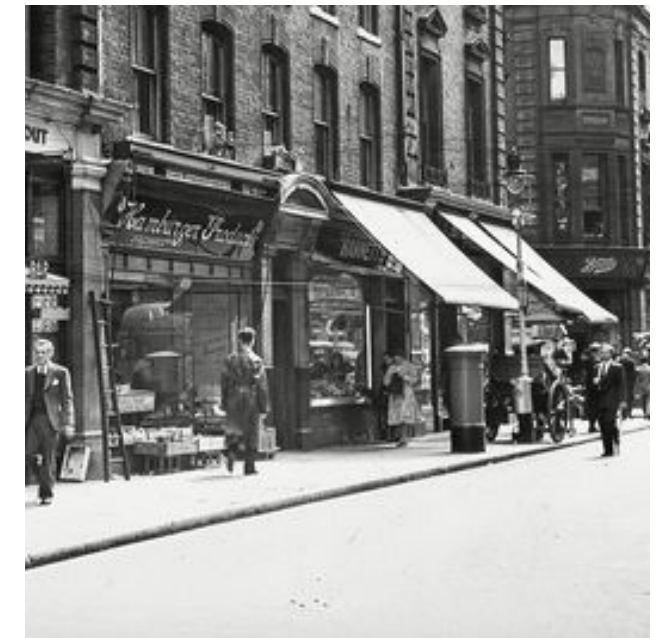
Fig. 114. London Victorian shop front with extended awning.
