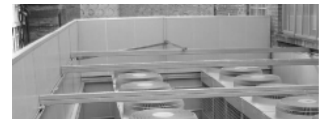
Fig. 146. Acoustic panels - screening to stop sound spreading.
