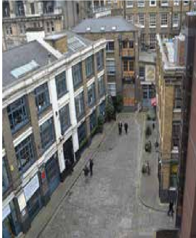
Fig. 123. View of Bleeding Heart Yard.
