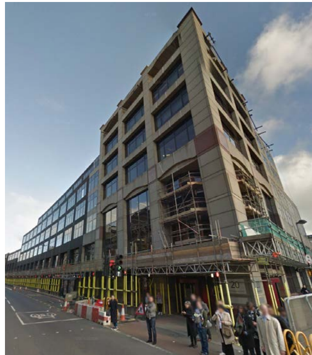
Fig. 116. 6 storey large commercial building on Farringdon Road.
