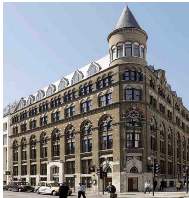
Fig. 118. 6 storey 25-27 Greville Street,
