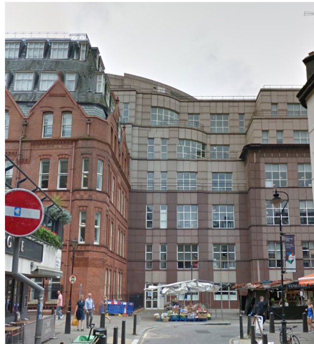
Fig. 120. 6 storey Prudential Building closing Greville Street.
