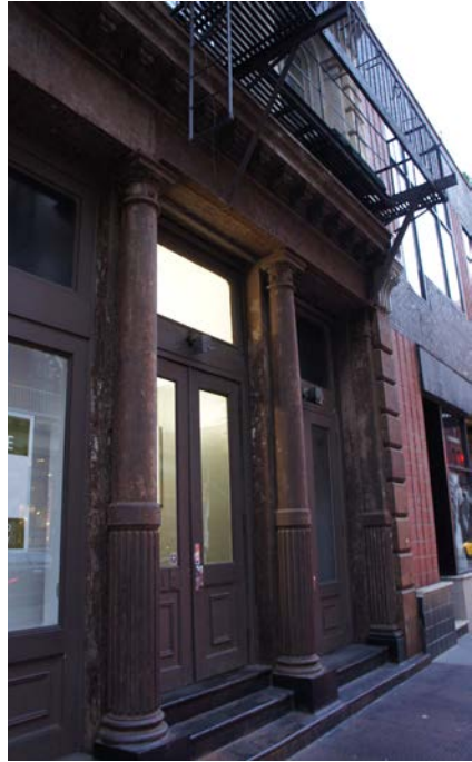
Fig. 59. Cast iron building facade, Soho, New York.
