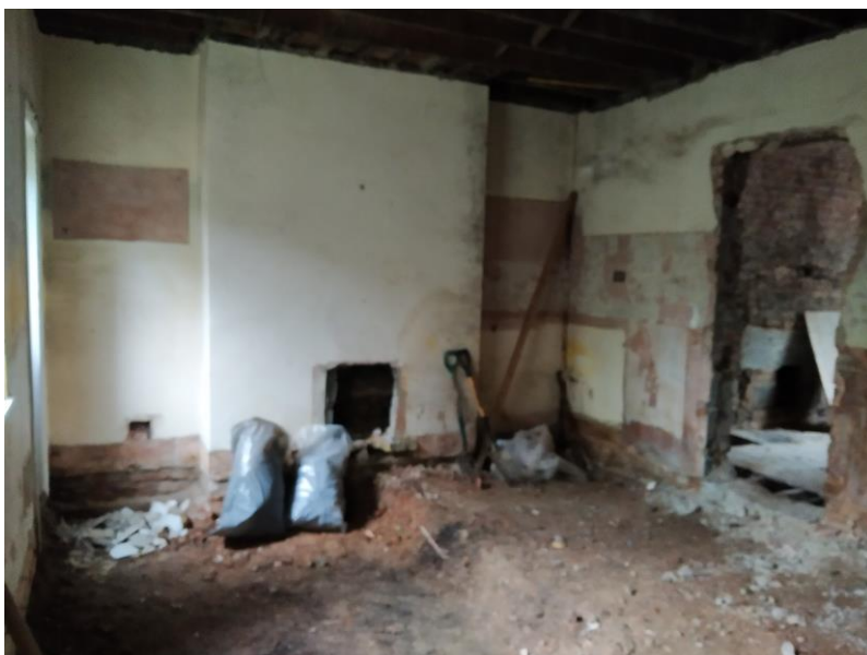
Photo 6: Foundation inspection pits have been completed
