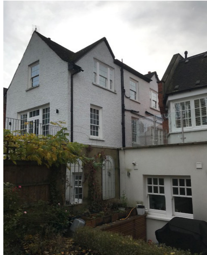
EXISTING BUILDING REAR VIEW LOOKING AT NEIGHBOUR BOUNDARY
