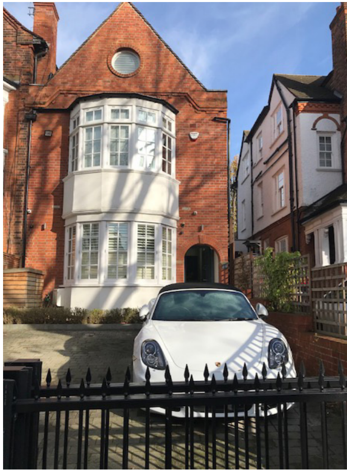
EXISTING BUILDING FRONT VIEW
