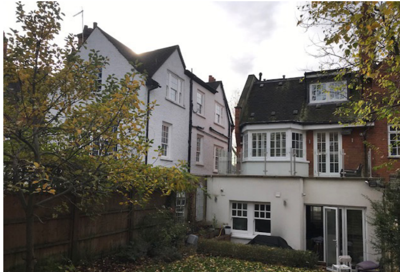
EXISTING BUILDING REAR VIEW
