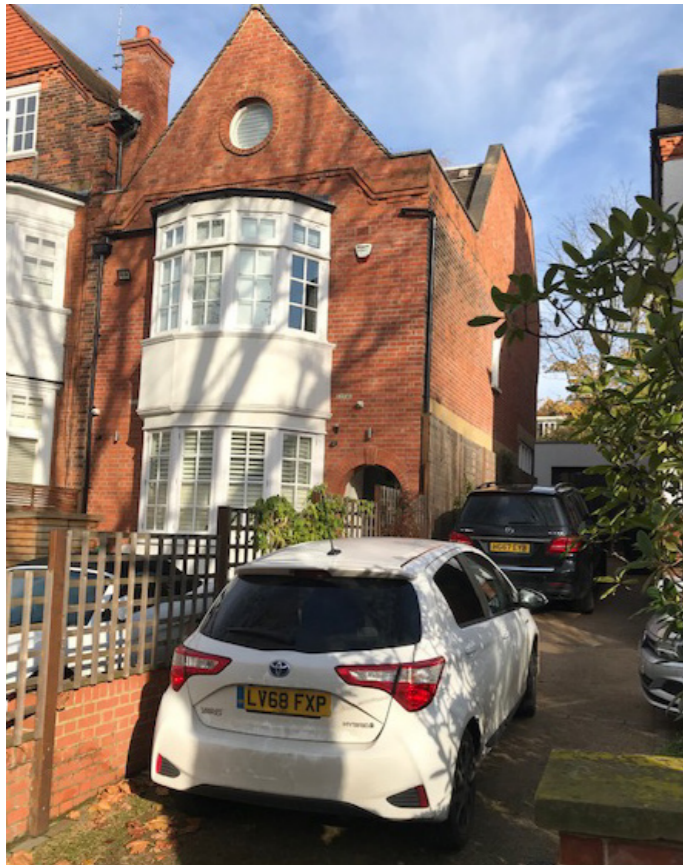
EXISTING BUILDING FRONT VIEW AT NEIGHBOUR SIDE BOUNDARY
