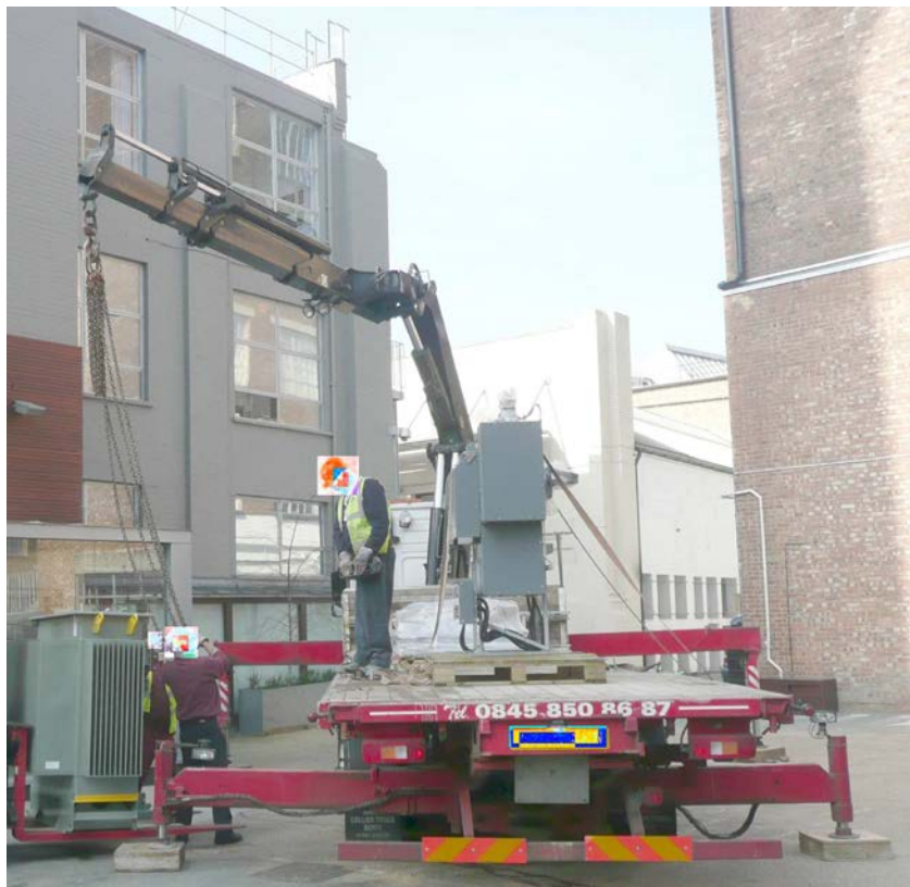
Photo 2: Example of plant delivery with 'out-riggers';
