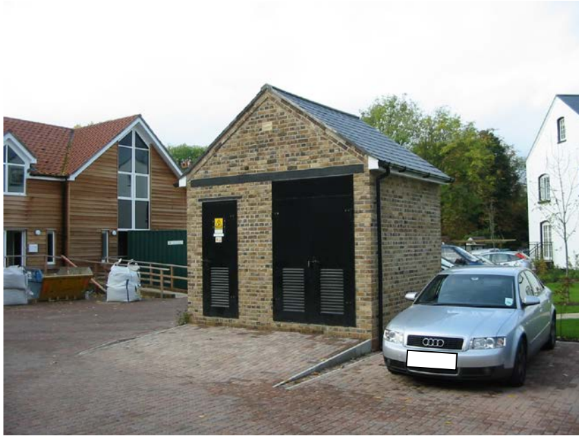
Photo 7: Substation with 'pitched' roof ~ Example 1;
