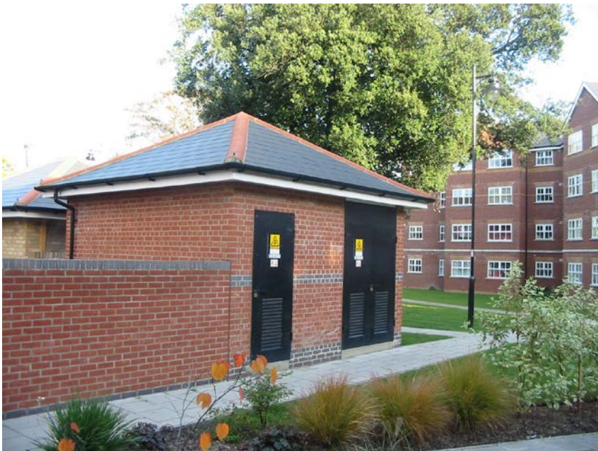
Photo 8: Substation with 'pitched' roof ~ Example 2;
