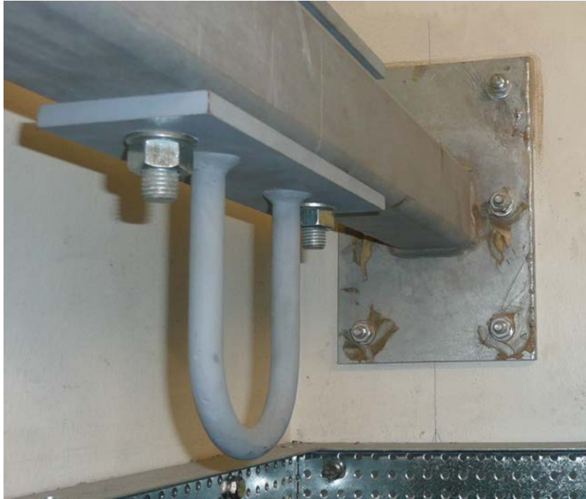
Photo 11: Example of 'Winching eye' for cable installation;
