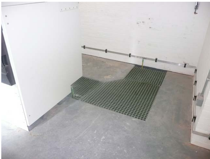
Photo 5: Example of 'Captrad' GRP floor gratings;
