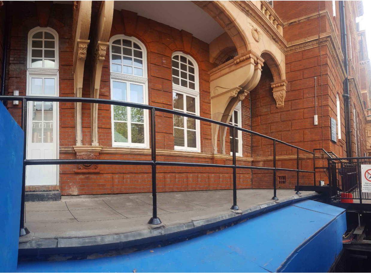
FLAT ROOF AFTER
