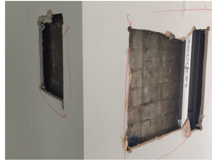
Strip out at wall with exposed brick
