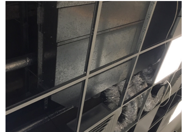
Existing HVAC services to the ceiling strip out
