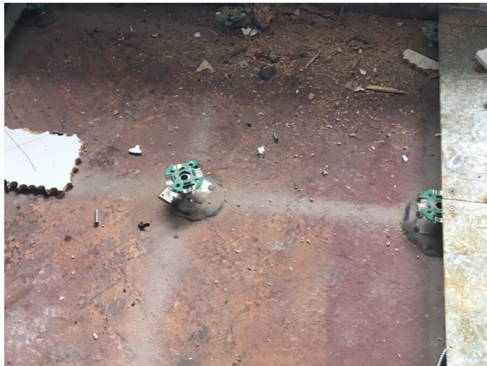
Strip out of flooring with indication of removed original parquet flooring
