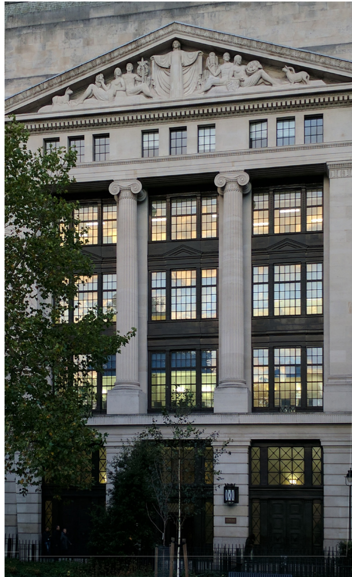
West facade central distyle-in-antis portico
