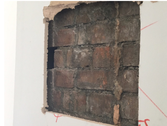
Strip out at wall with indication of removed panelling
