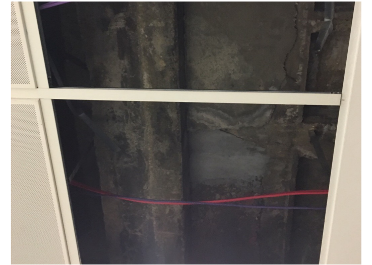
Strip out at ceiling indicating 2003 refurbishment with ribbed concrete slab
