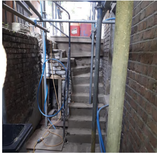
EXISTING CONDITION OF STAIRCASES
