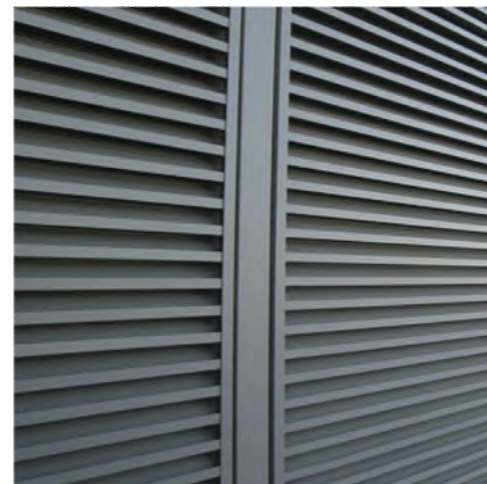
Aluminium Power Coated Louvers RAL colour 7043 For Acoustic Spec refer to Full Planning Application PP-08264900
