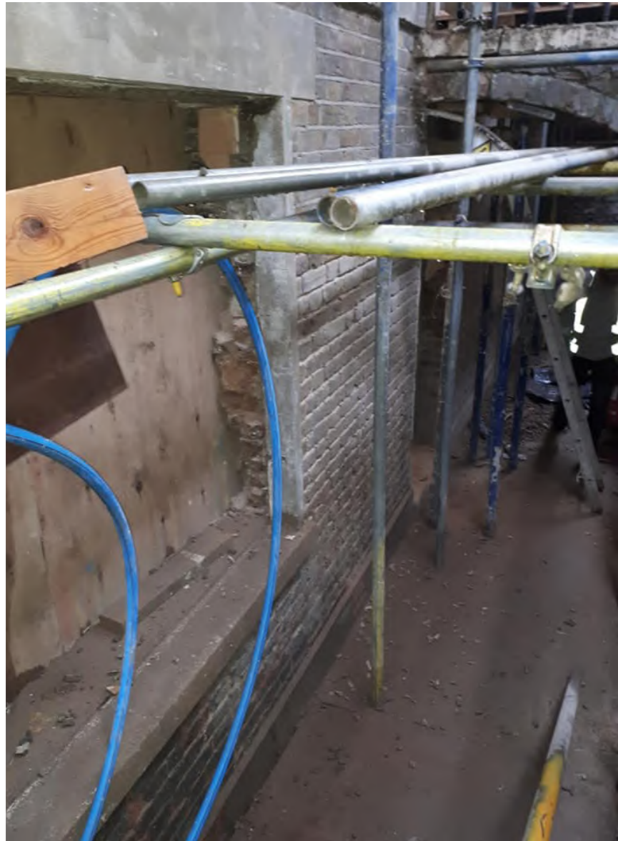
PHOTO 1. PHOTO OF THE EXISTING FULL HEIGHT OPENING
