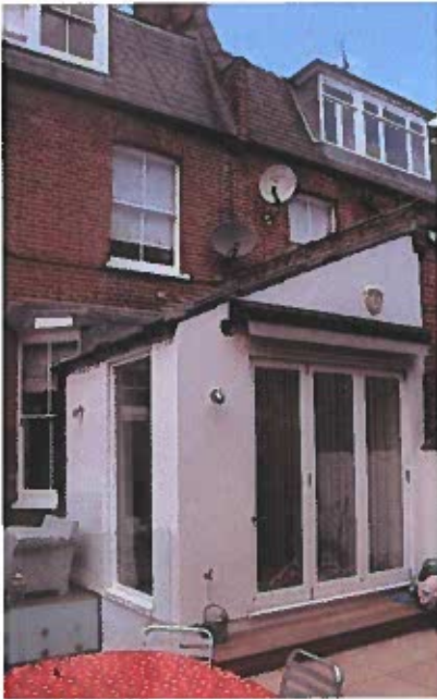
Rear (east) elevation and outrigger extension. The canted bay window, seen on the left, will be removed as part of the proposal.
