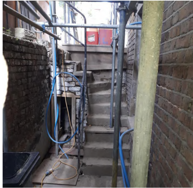
EXISTING CONDITION OF STAIRCASES
