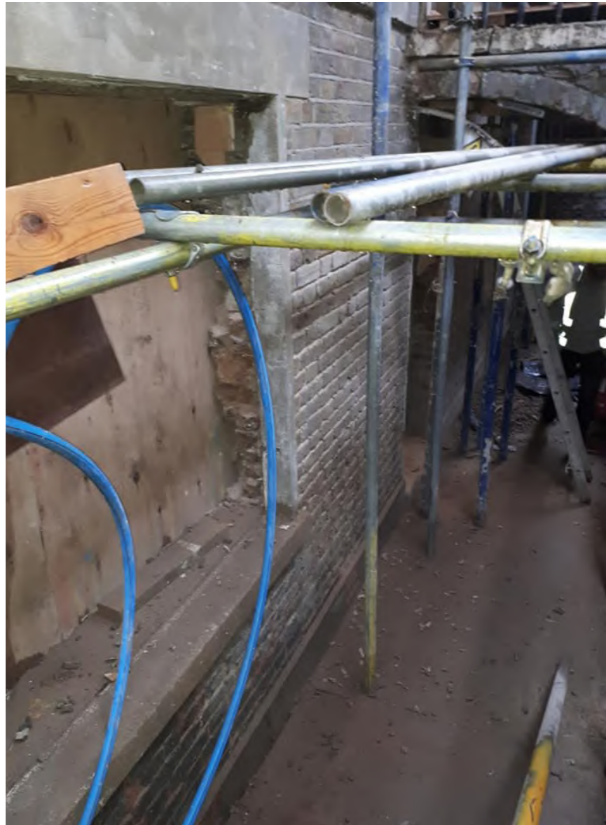
PHOTO 1. PHOTO OF THE EXISTING FULL HEIGHT OPENING
