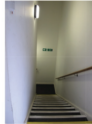
12 First Floor Staircase
