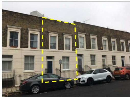
Fig.1 16 Pakenham Street (front) and rear - right
