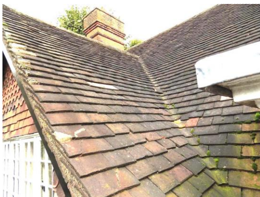
Broken and slipped tiles to roof 6
