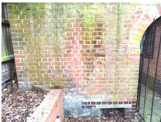
Cracking to wall to west boundary
