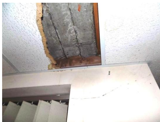
Damp to lower floor of extension
