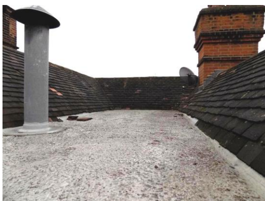
Coated flat roof 9 over lift
