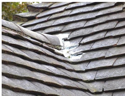
Coating patch to rear of roof 6 dormer
