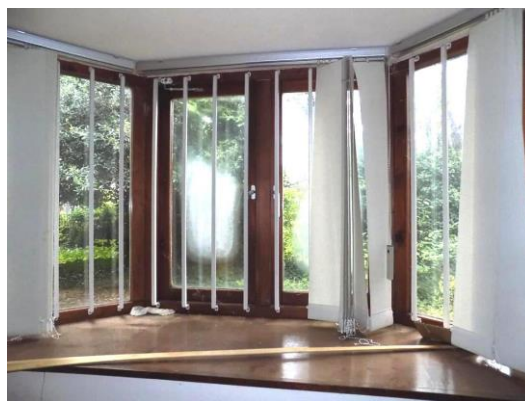
Failed double glazed units to extension
