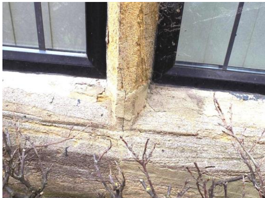
Poorly repaired cills and mullion
