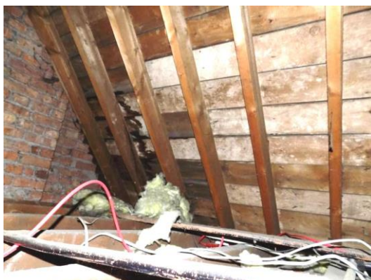
Damp stains to chimney to roof 15/16
