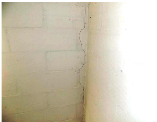
Cracking to lower floor of extension
