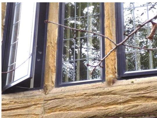
Eroded stone mullions
