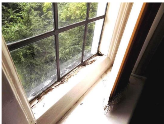
Internal decay to cill
