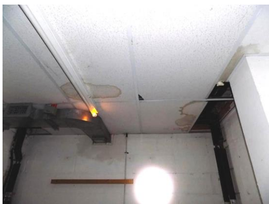
Damp to lower floor of extension
