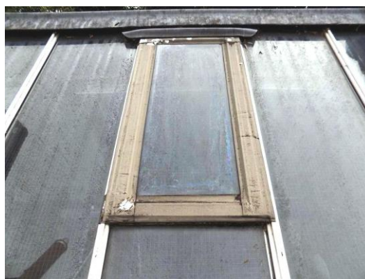
Flashband repair to glazed roof
