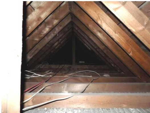
No insulation to roof void 5
