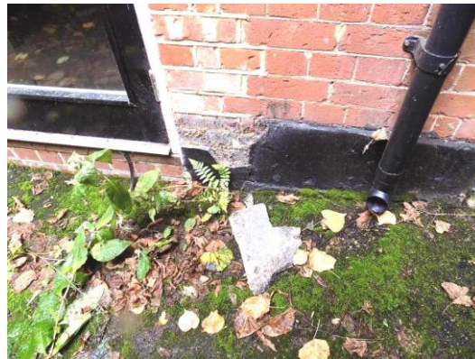
Failed render plinth to north elevation
