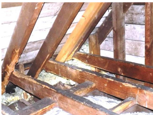
Squirrel damage in roof 21
