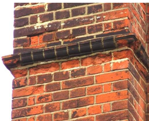
Spalling brick to chimney stack 4
