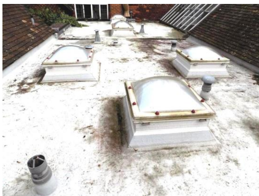
Coated flat roof to extension
