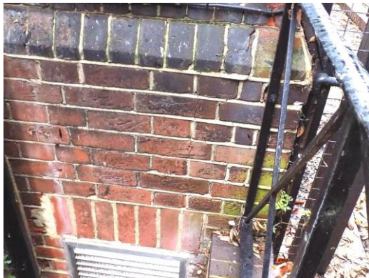
Cracking to side of south bay window
