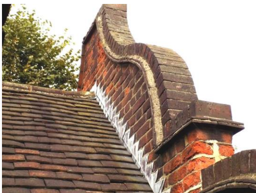
Eroded pointing and spalling to east elevation
