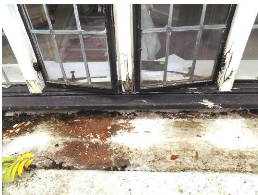
Decay to staircase window
