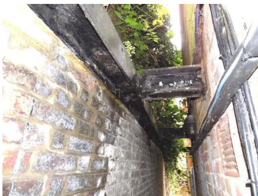
Steel beams and braces to north wall
