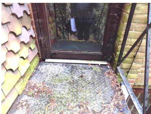
Decay to fire door to extension
