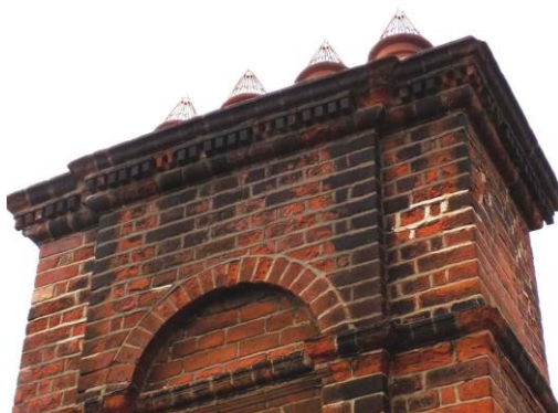
Spalling brick to chimney stack 4
