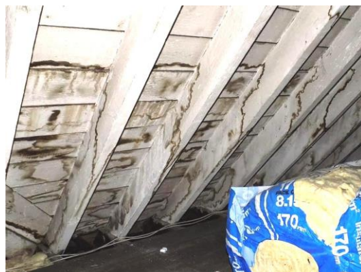
Damp staining below raised flat roof 9
