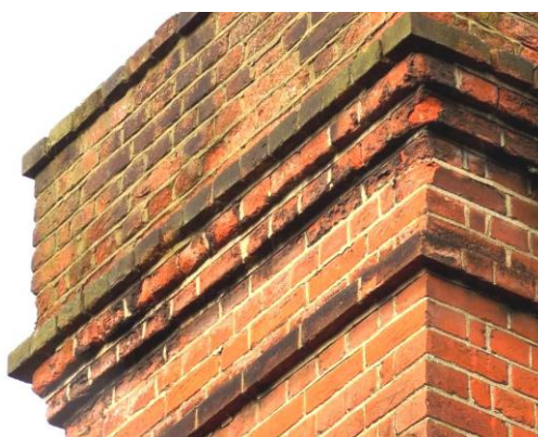
Spalling to chimney stack 6
