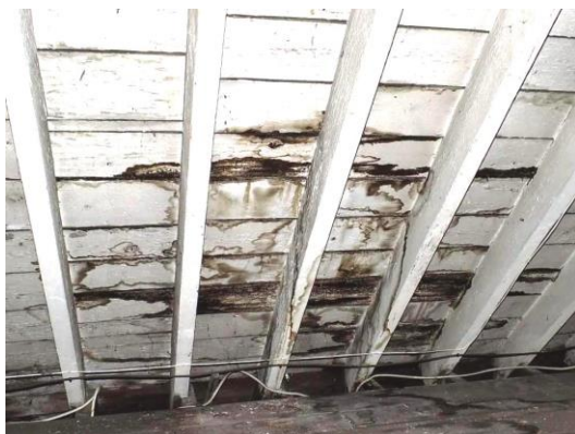
Damp staining around chimney 4
