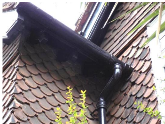
Replacement cast iron gutters and pipes
