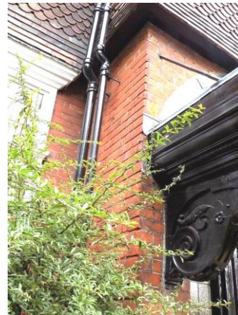
Eroded pointing to side of south door
