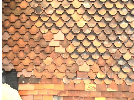
Patches of incorrect tiles
