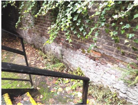
Spalling to north boundary wall
