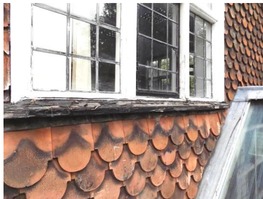
Decay to first floor west window
