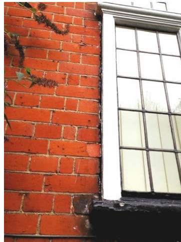
Missing frame sealant/pointing
