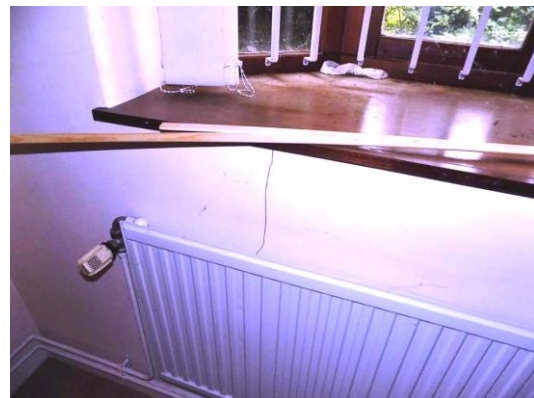
Cracking below south window in extension
