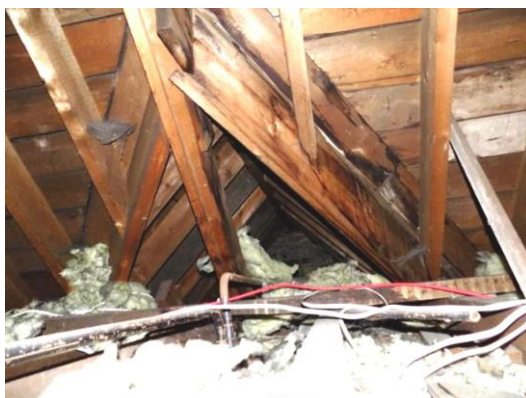
Damp stains to raised gable to roof 16
