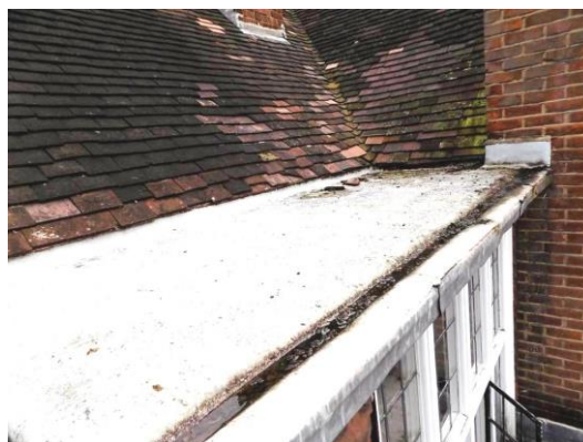
Coated flat roof to bay window
