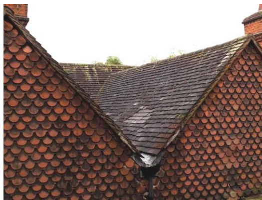
Valley gutter above staining
