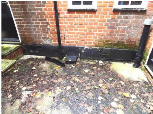
Render plinth to north elevation
