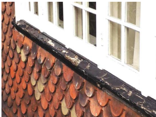
Decay to first floor west window
