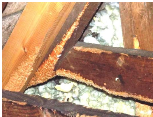
Squirrel damage in roof 21
