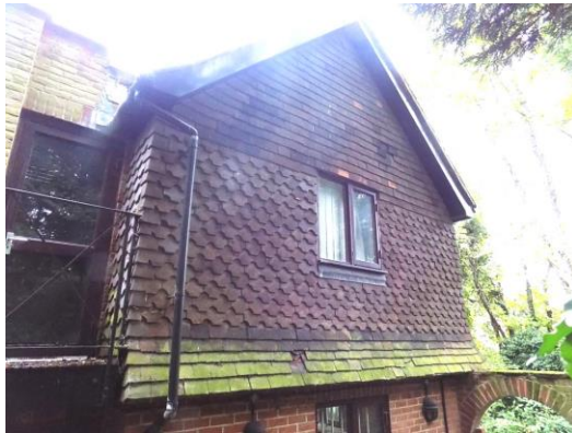
Missing tiles to extension
