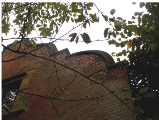
Eroded pointing and spalling to east elevation
