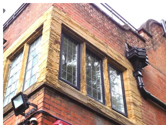
Eroded and redressed stone
