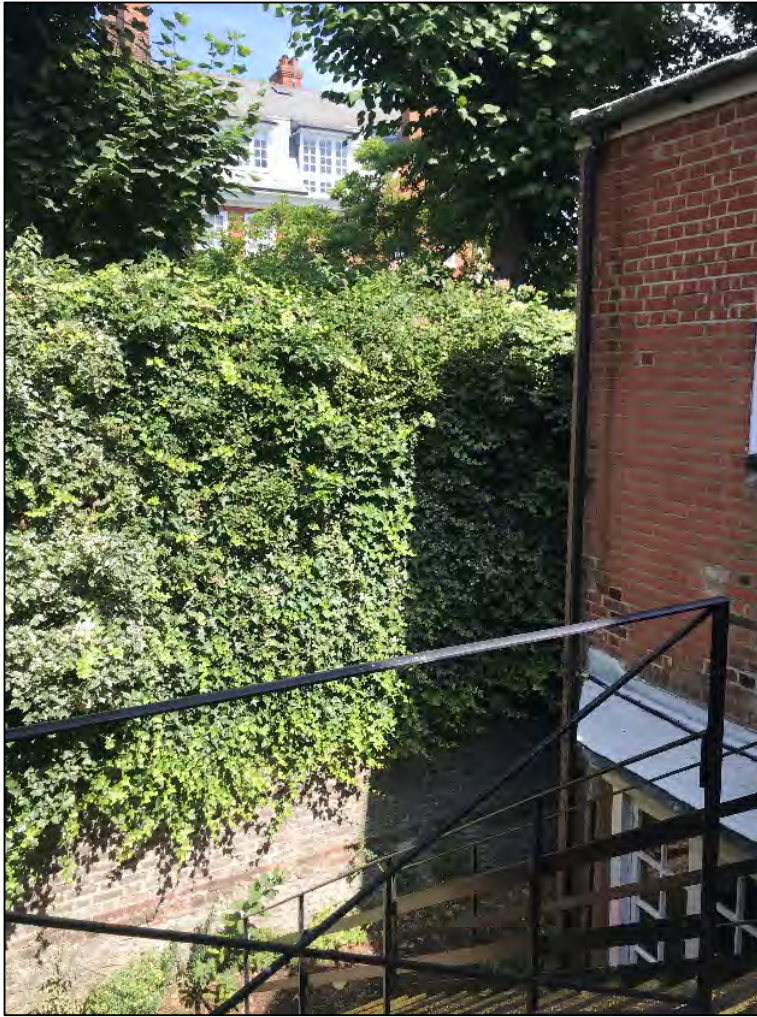
Photograph 3: Level change and retaining structure between application site and G6
