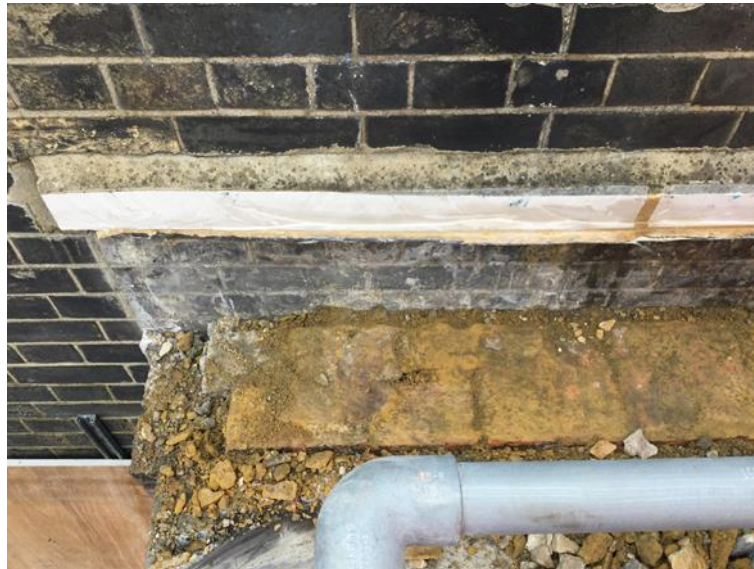
Figure 14. Walkden House coping stones embedded into the RCGP northern elevation
