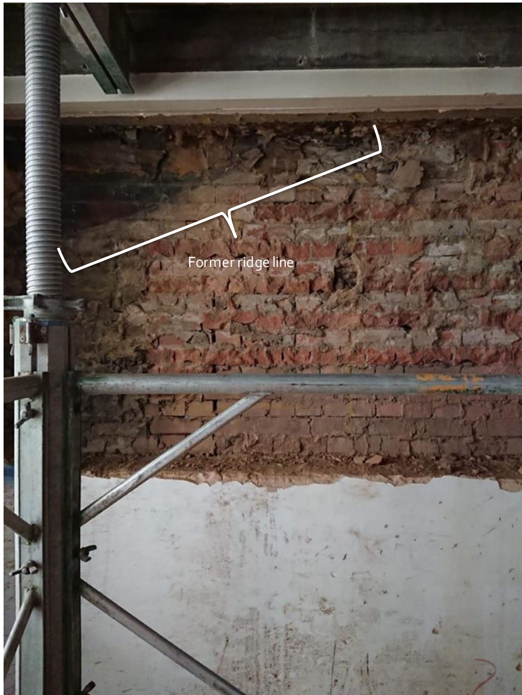
Figure 8. The ridge line of former 19th century terraces visible on the RCGP northern elevation, revealed behind the second storey brick infill of Walkden House (Mott MacDonald, 2019)
