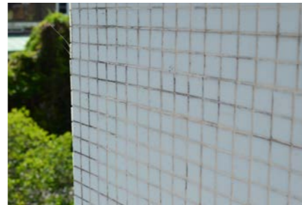
Existing mosaic facade
