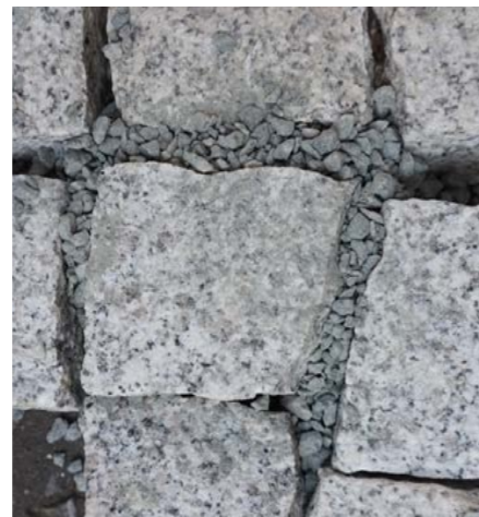
Small unit granite setts with grit joints
