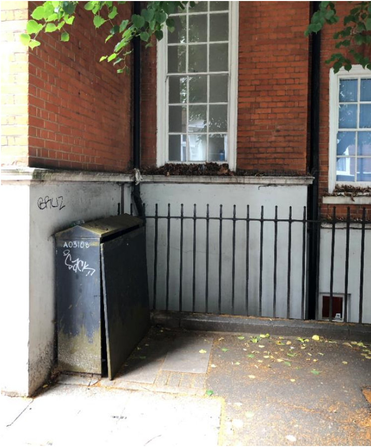
Figure 9 – View of lightwell from pavement level
