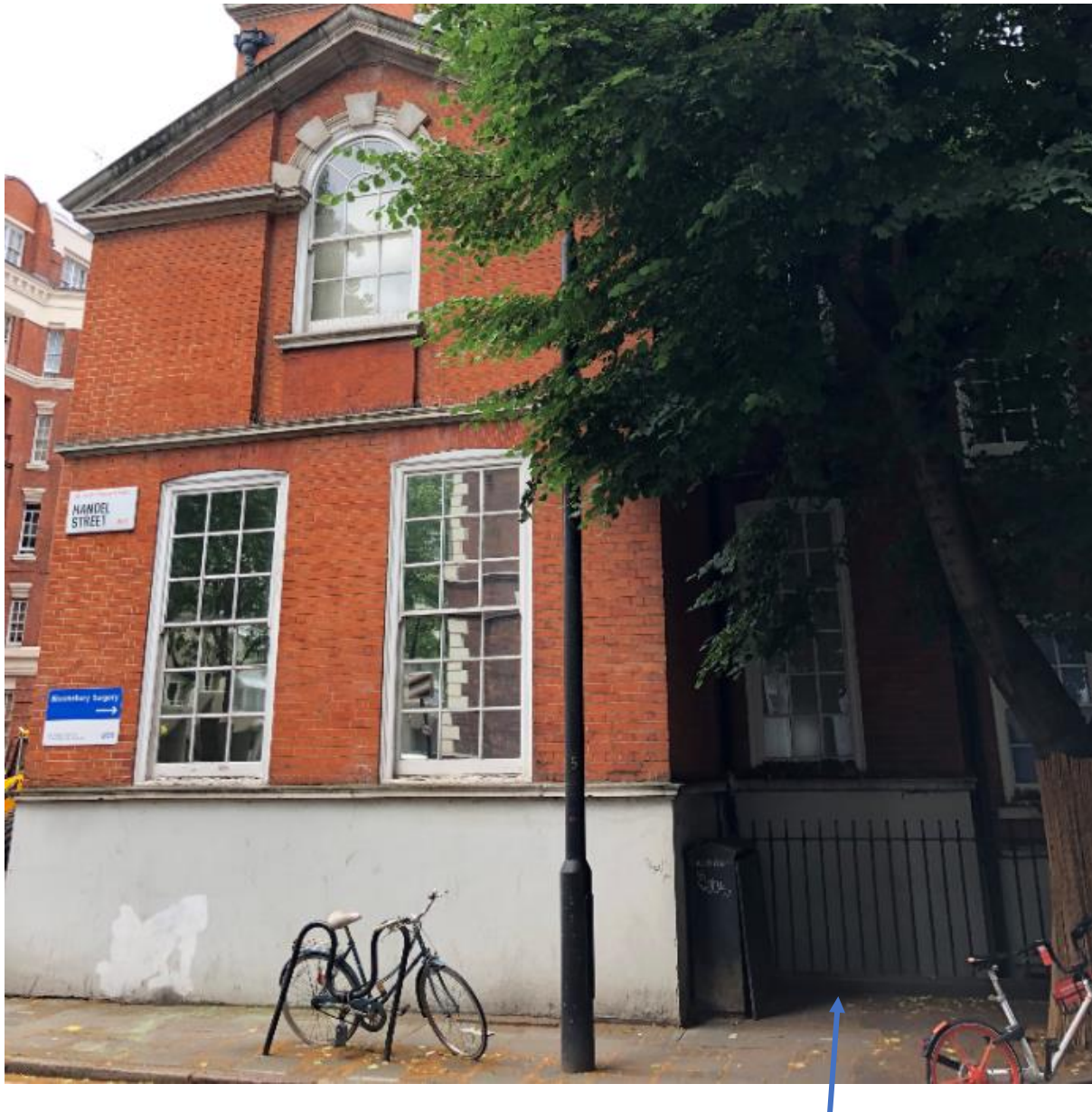
Figure 12 – South-western corner of Hunter Street, including the lightwell in which work will be accommodated.
