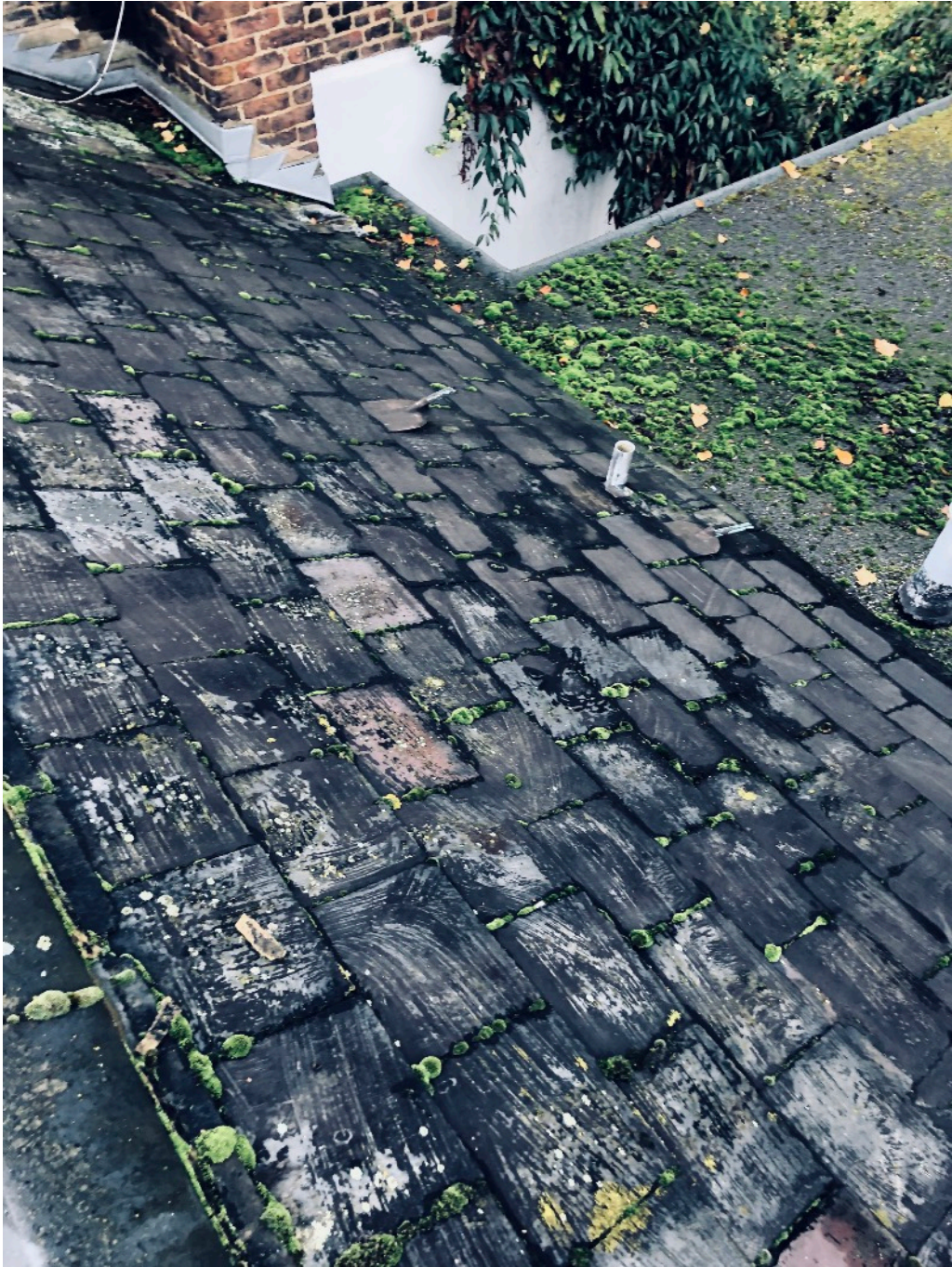
rear roof slope
