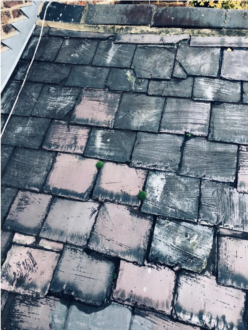
detail of slates
