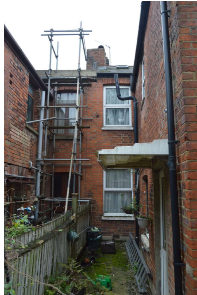
Side Passage looking West
