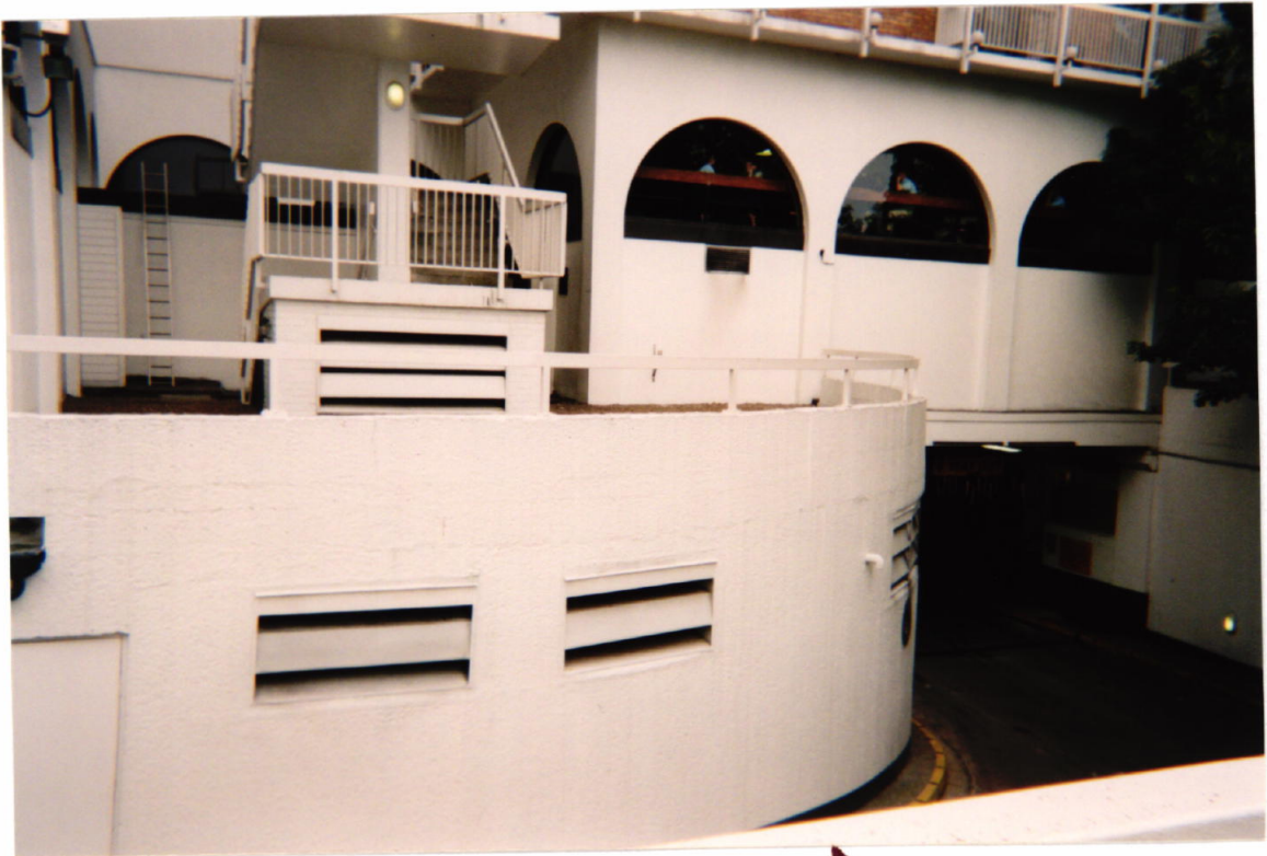
FRONT ELEVATION AND DELIVERY BAY ENTRANCE ↗
