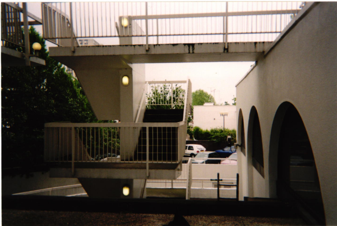
STANDING ON EXISTING FLAT ROOF LOOKING OUT. ↗
