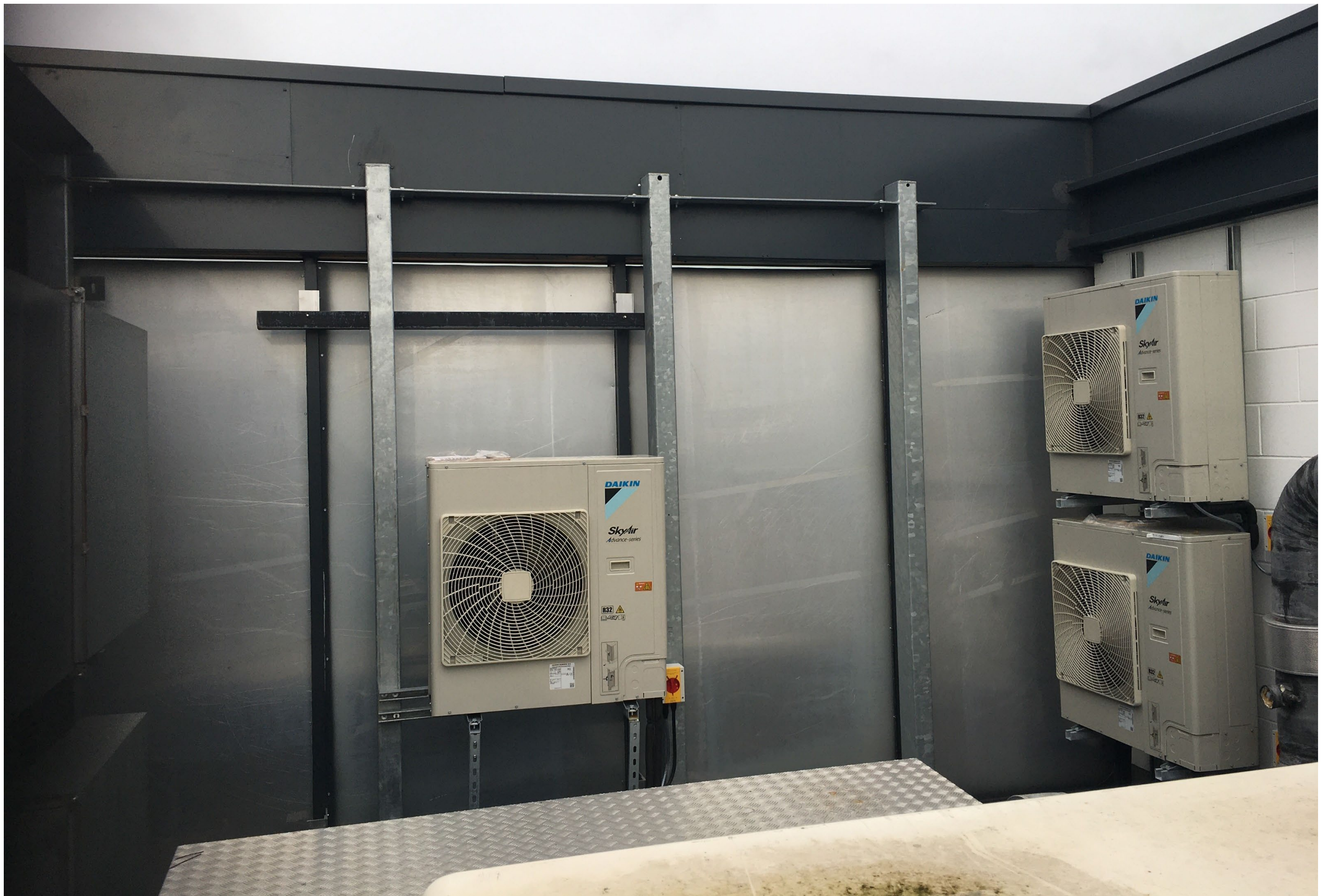
SSP - Jamestown Wharf: Planning Application Site Photo (Existing Screened Plant Enclosure Space for External Condensers)
