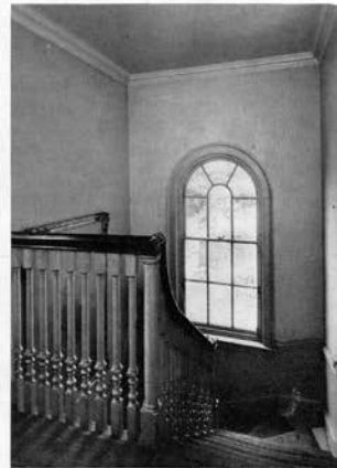
18.—THE GEORGIAN STAIRCASE
