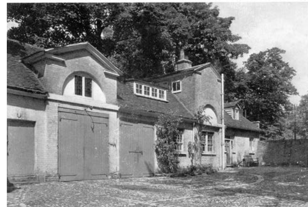
Historic photograph from 1949, showing the front of the stable block and gardeners accommodation (111) prior to conversion and listing in 1950
