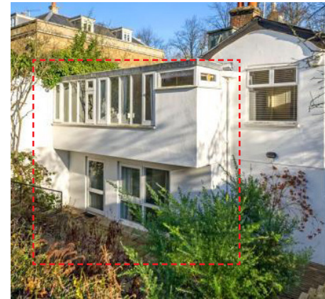
Rear north extension
