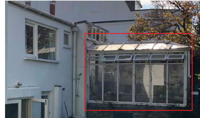
Photograph of existing uPVC greenhouse to be removed
