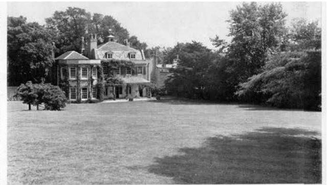
13.—LOOKING DOWN ON THE HOUSE FROM ACROSS THE LAWN. The modern wing is on the left
