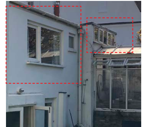
Boxback extension and flat roof of south transept
