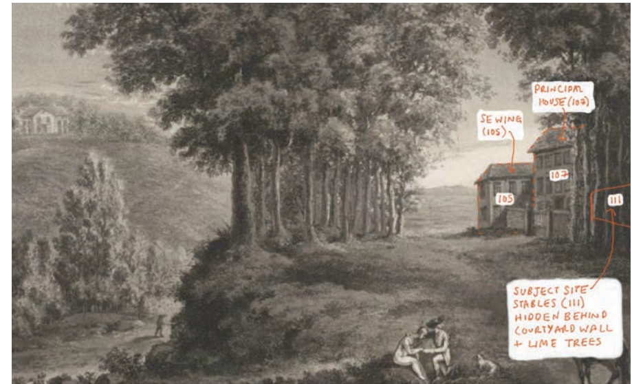
Front View of Frognal Grove from lime avenue (1790)
