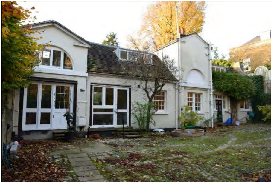
Plate 4: Southeast elevation of 111 Frognal, looking northwest
