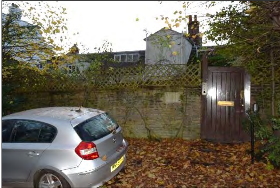
Plate 5: Boundary wall of 111 Frognal with house beyond, looking west-northwest
