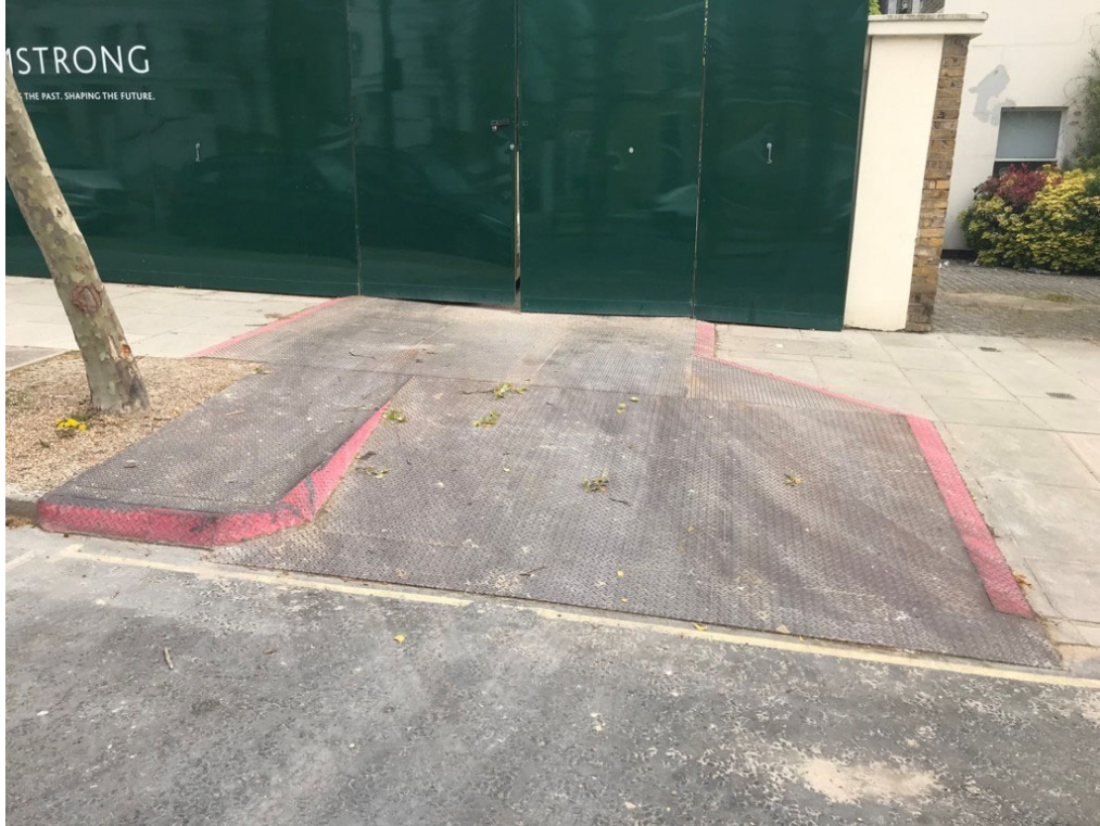
Photograph 1: Example of ground protection using steel checker plate
