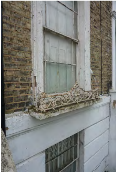
Example of original decorative baluster
