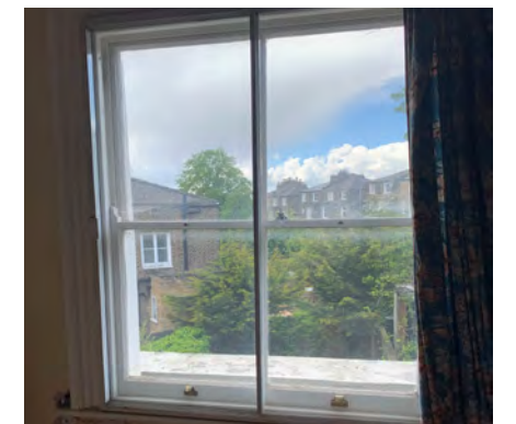
Modern windowreplacement to rear
