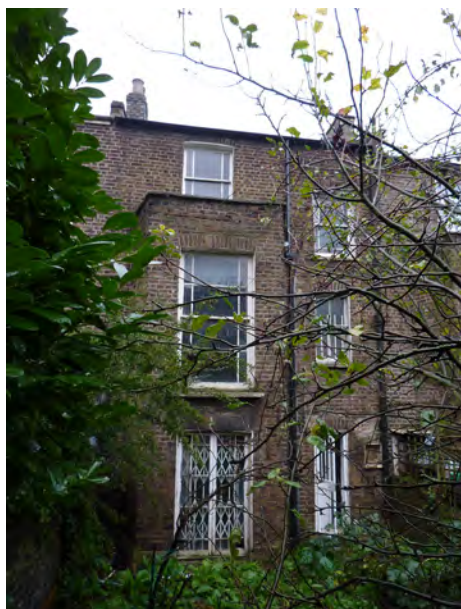
Original rear elevation at 6 St Pauls Crescent
