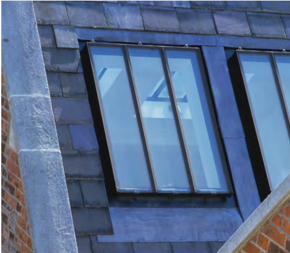
Conservation rooflights flush with roof finishes.
