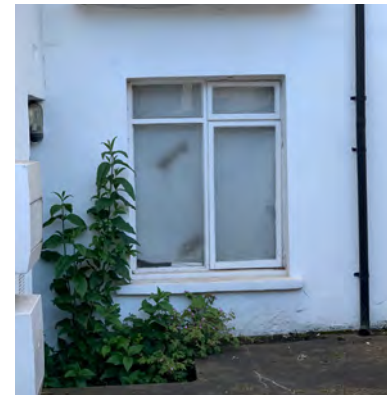
Typical replacement casement window
