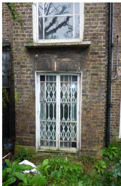
Original french doors to the garden at 6 St Pauls Crescent
