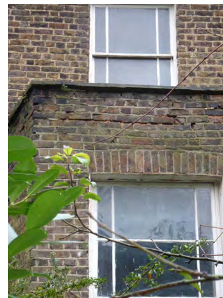
Original stone capped balcony to bay window.
