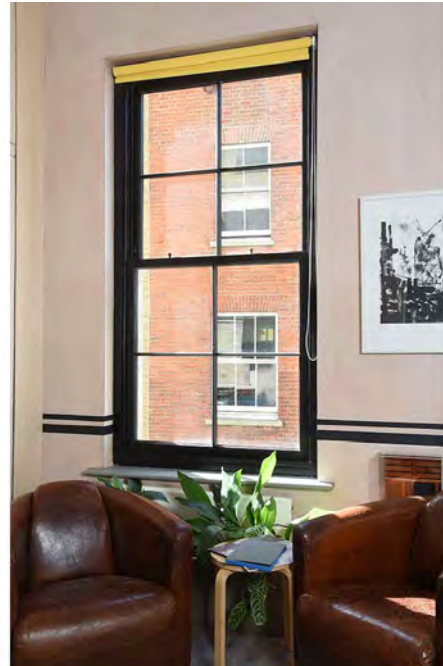
Example double glazed sliding sash window
