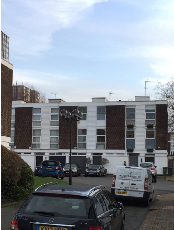
View of existing roof boxes from Hawtrey Road.
