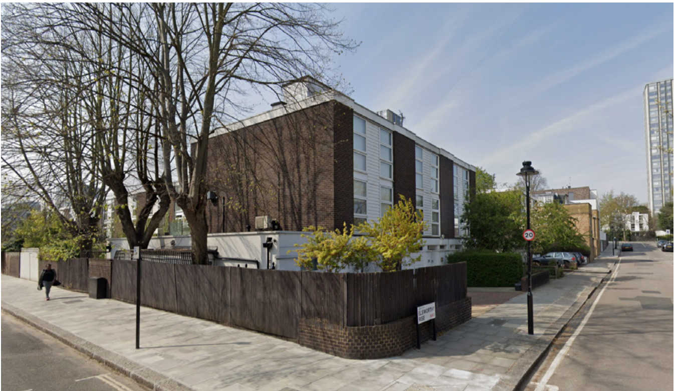
View of existing roof boxes from Elworthy Rise.
