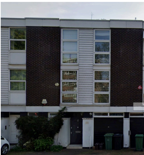
View of 99 Fellows Road from Fellows Road
