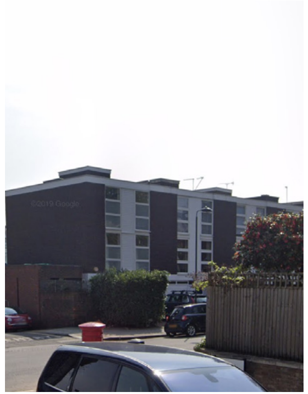
View of existing roof boxes from Fellows Road.
