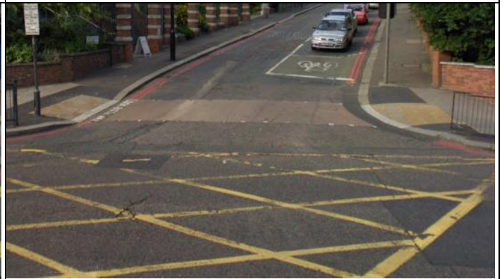
June 2008 Poor junction state, subsidence & frequent patching, some due to water mains leaking & bursts
