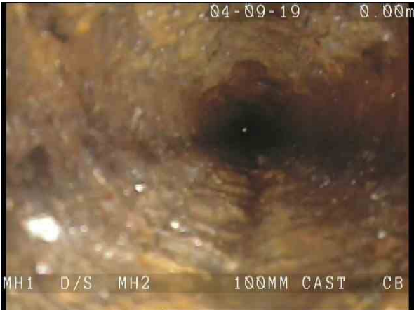
MH1X_697d6ba7-1a86-43ea-9b00-4985f68a1723_20190906_095824_558.jpg, 00:00:06, 0.10 m Attached deposits, encrustation from 12 o'clock to 12 o'clock, 5% cross-sectional area loss, start
