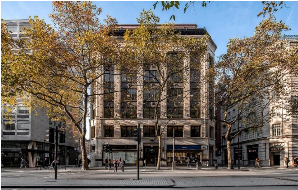
Figure 1: Kodak House (Source: Google Maps, 2019)
