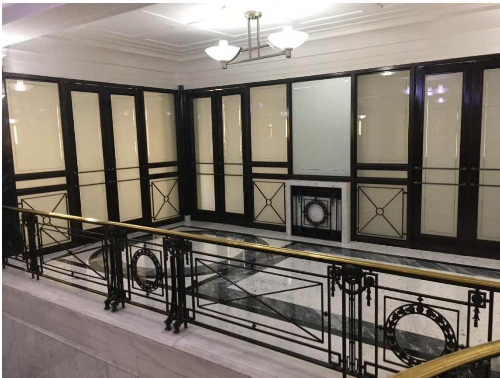
Figure 29 Interior of the principal entry hall at first floor level (2019. Note repositioned elements of the balustrade and modern glazed screening to the board room.
