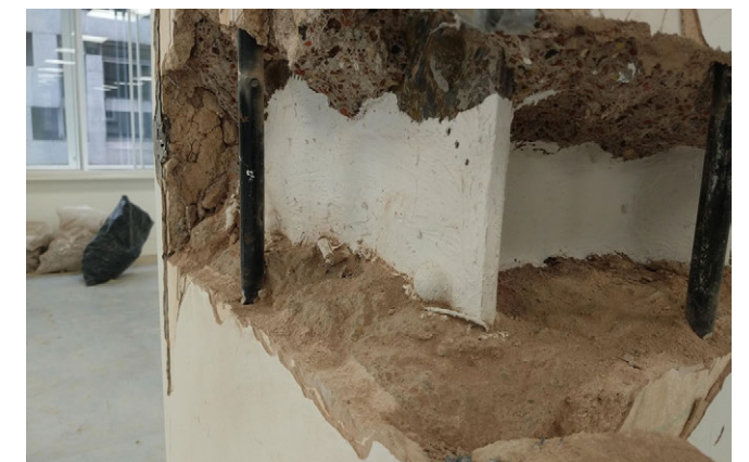
Column With Rivetted Plates
