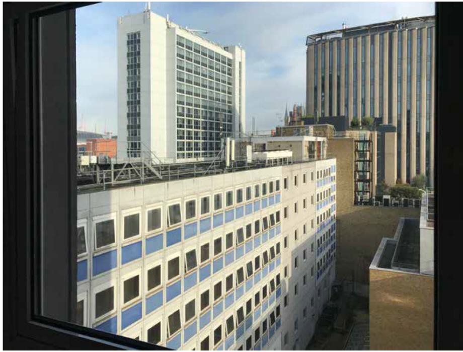
Existing view from a habitable room in Somerton House
