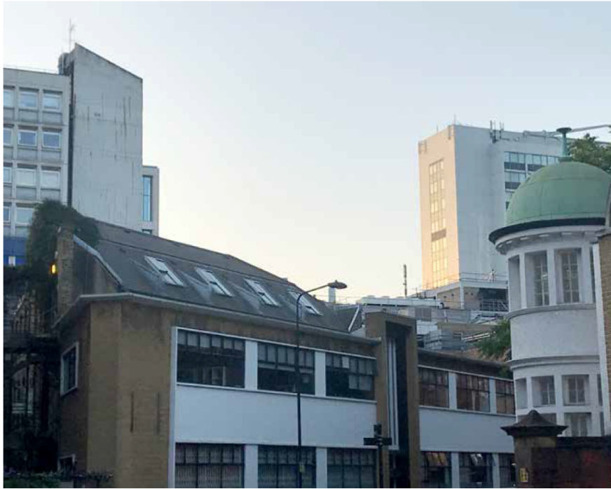
Existing view from Burton Street in Bloomsbury Conservation Area
